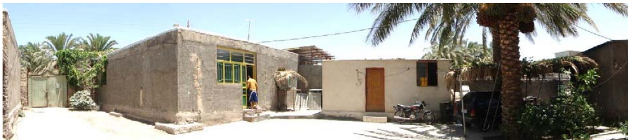
Figure 2: Temporary units made of masonry materials became extra rooms after reconstruction
